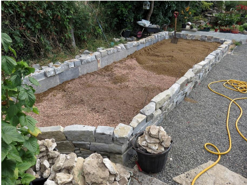
Bulb bed under construction.
